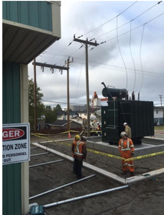
Transformer installation on the GND site
